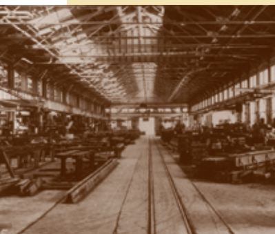
Bethlehem Steel Company Foundry, 1945.
